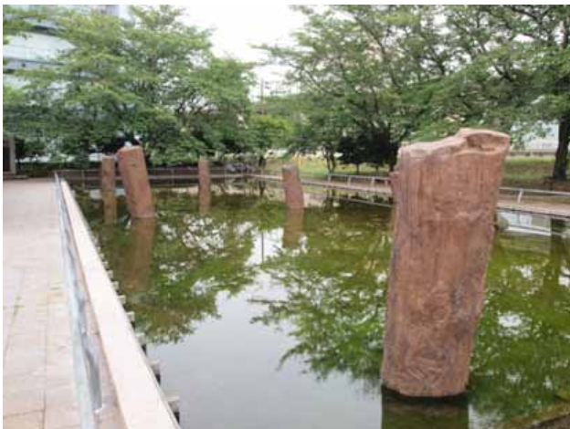
図6 地盤の液状化で出現した旧相模川橋脚の遺構 Fig. 6 The relic of piers of old bridge in Kamakura period emerging with the soil liquefaction due to earthquake.
