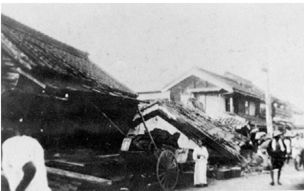
図 3-a. 関東地震で民家が倒壊した本町通りの写真 Fig.3-a The photo of damaged houses by the Kanto Earthquake in the “Honmachi avenue”.
