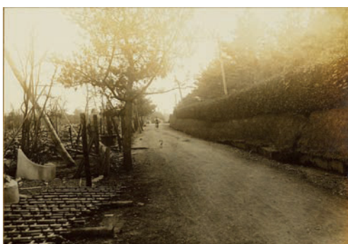
写真11 正門付近外構土塁(震災後) Photo11 The earthen wall near the main gate (after the earthquake)
