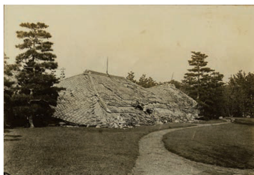
写真 8 御座所(震災後) Photo8 The princess room (after the earthquake)
