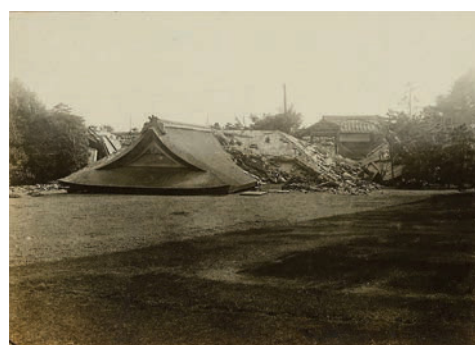
写真 6 御車寄(震災後) Photo6 The carriage (after the earthquake)
