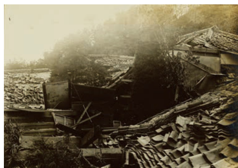
写真12 臣下昇降口(震災後) Photo12 The subjects' doorway (after the earthquake)
