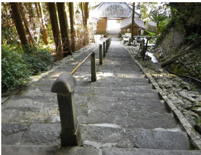
図5 青龍寺 手洗場より下の石段 津波後、新しく造り替えられ石の表面に凹凸が残る。 Fig.5 Stone steps below the hand washing place at the Shoryuji, temple 36. Since it was rebuilt after the 1707 Hoei tsunami, the surface of the stone steps remains uneven.
