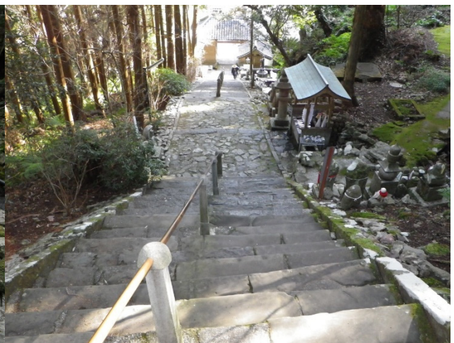
図6 青龍寺 手洗場より上の石段 数百年以上の年月踏み締められ平滑である。 Fig.6 Stone steps above the hand washing place at the Shoryuji, temple 36. Since it they have been trampled over for hundreds of years, the surface of the stone steps is smooth.
